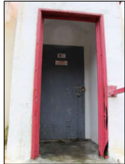
Photograph 11 – Deteriorated wood frame jamb
