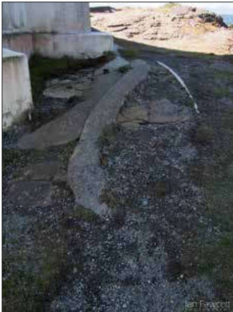
Image 24 (left): previous above-ground asphalt covering - not to code
