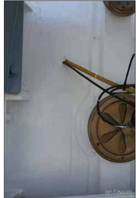
Image 85 (right): cables re-routed through new holes/couplings in lantern room wall adjacent to vent
