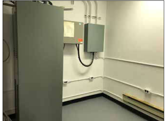
Images 122 (top left) and 123 (bottom left):: showing condition of interior walls and floor - note mould in corner and wrinkling along bottom
