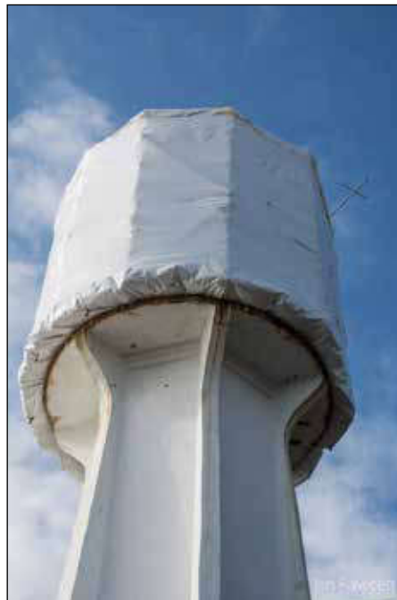
Image 44, 45 and 46: scaffolding (in process) and completed sheathing erected around lantern room
