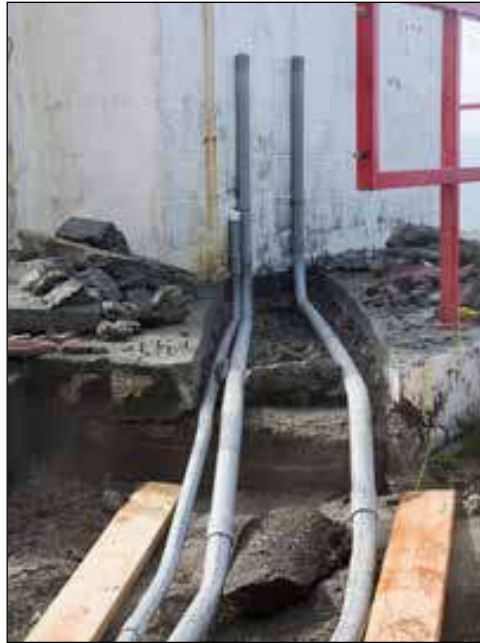
Image 27 (top left): forms for concrete conduit cover
