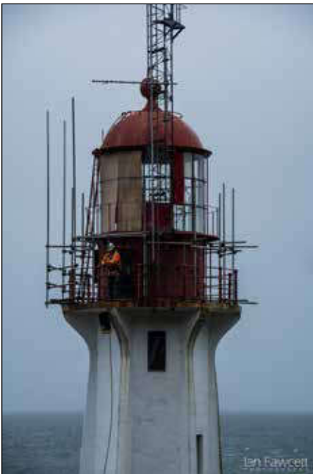
Image 44, 45 and 46: scaffolding (in process) and completed sheathing erected around lantern room
