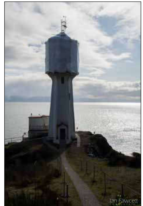
Image 44, 45 and 46: scaffolding (in process) and completed sheathing erected around lantern room
