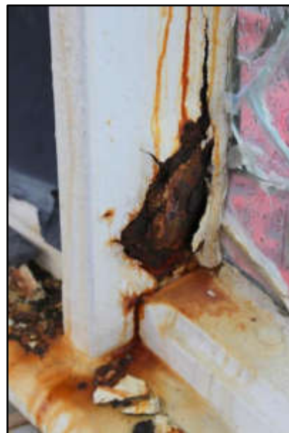
Photograph 6 – Moisture ingress and acute corrosion at the base of the support tube
