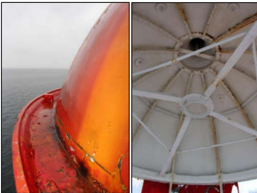
Photographs 7 & 8 – Discoloured exterior paint and corroding interior roof structure
