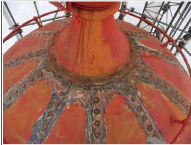
Image 60 (top left): weather vane showing corrosion and damage,
