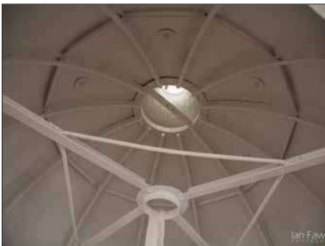
Image 74 and 75 (top row): original condition of lantern room interior, showing some corrosion
