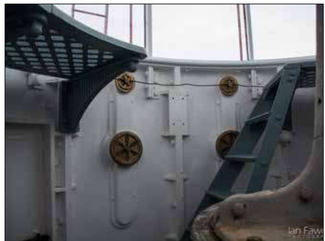
Image 74 and 75 (top row): original condition of lantern room interior, showing some corrosion
